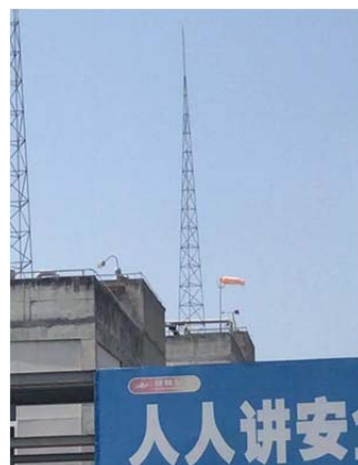
车间楼顶风向仪
