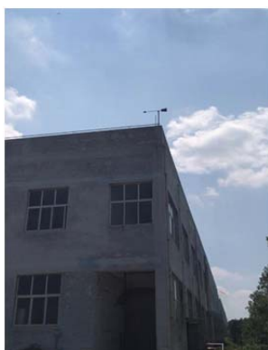
车间楼顶风向仪
